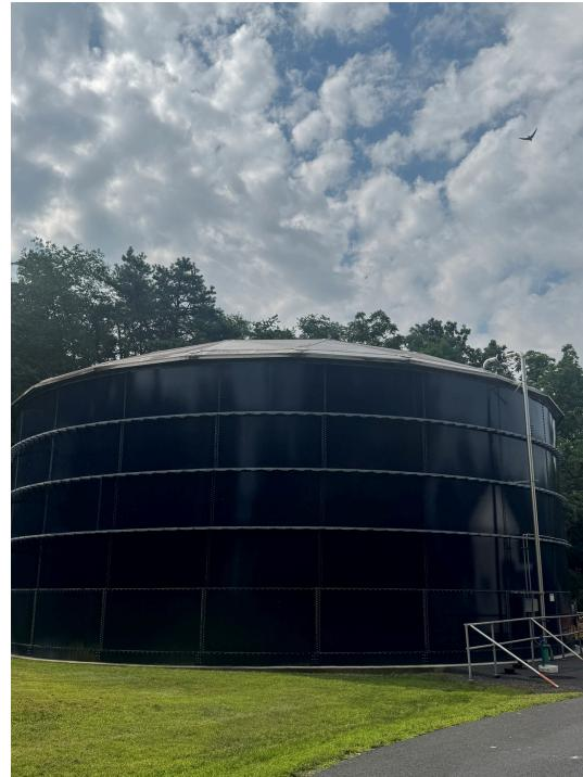
This is a biosolids storage tank! This is the final resting place before the sludge is pumped out and spread on fields. Our future sludge press will make this process more environmentally friendly and efficient.
